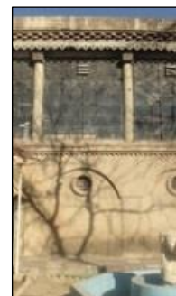
Combining old and modern style in the facade (after restoration)
