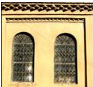
Merge elements from several different styles (after restoration).
